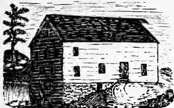
Old Mill at Hibernia.
